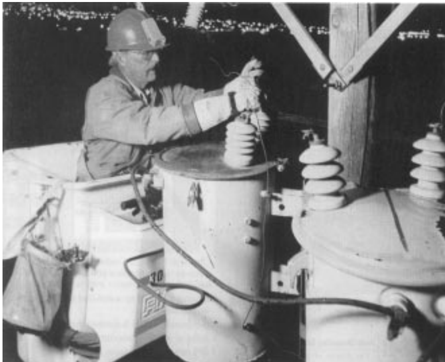
1. Conventional winter coveralls , known in the trade as Carhart’s, are preferred by many line workers and provide good protection form electric arcs, but both the shell and the non-flame-resistant polyester fill could ignite under some arc conditions
